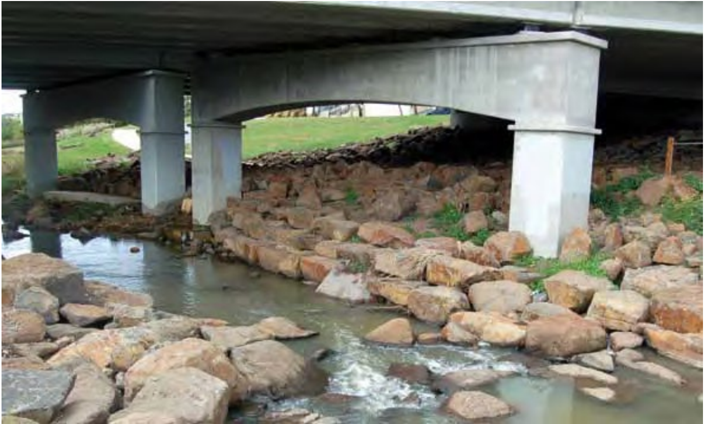
Figure 2 - exemplary rock work beneath a bridge with piers including provision for low flow maintenance
