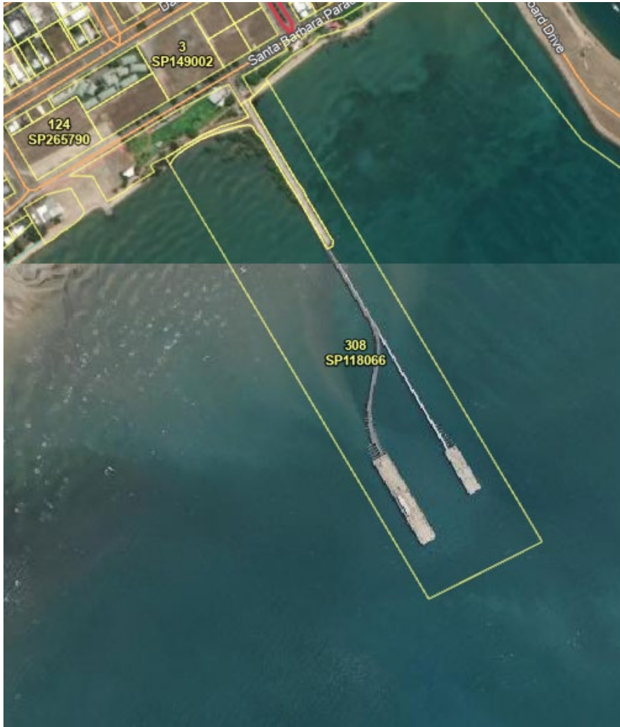
Figure A – Investigation Site
