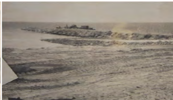
Plate 6: Reconstruction works, rockfill and barge hardstand (NAA)
