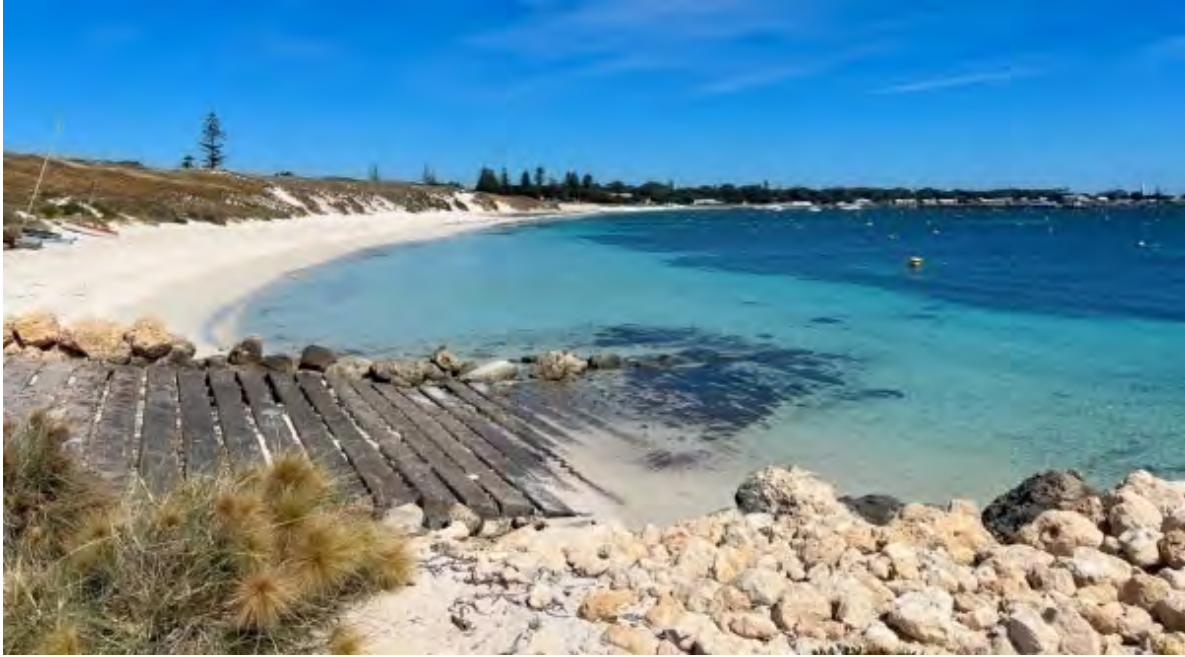
Plate 9: Public boat ramp at the Army Groyne
