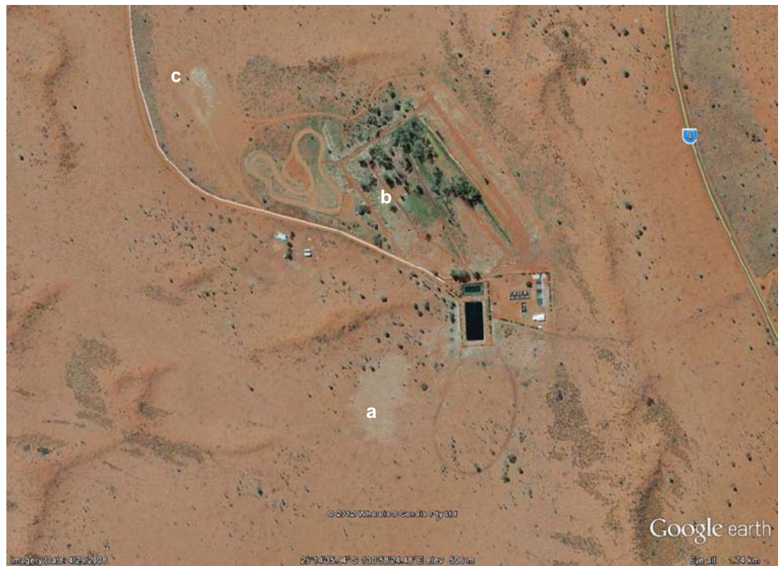
Figure A26: Yulara Wastewater Treatment Plant
