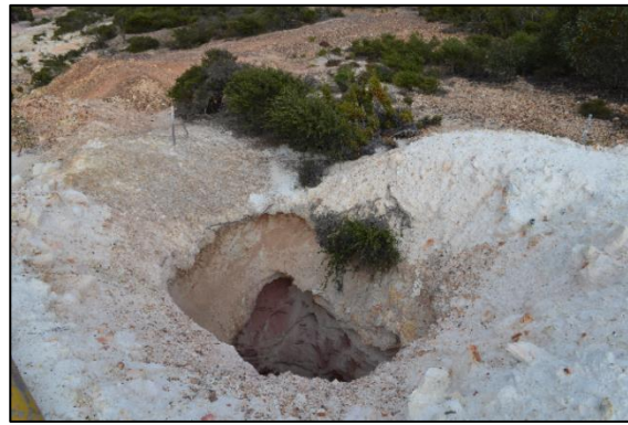
Plate 2: Unstable shafts in the Kundip mining area
