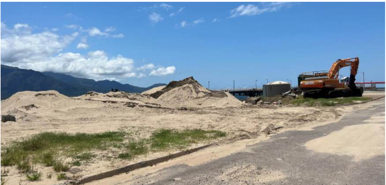
Figure 4-10 Dredge sand stockpiling at Lucinda Barge Ramp
