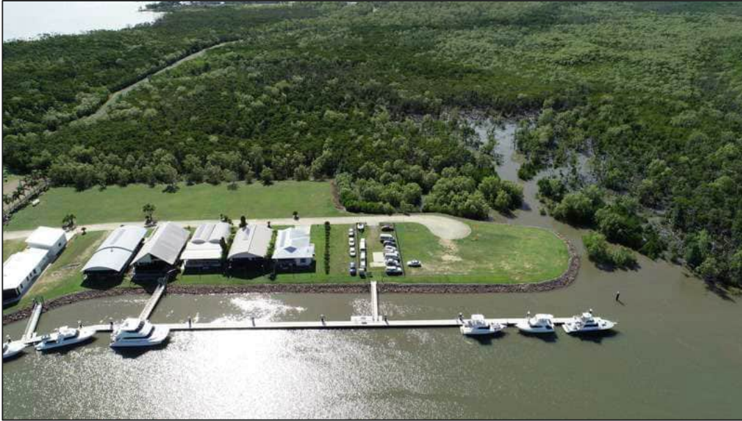
Figure 15: Retaining wall in Dungeness Enterprise Channel.
