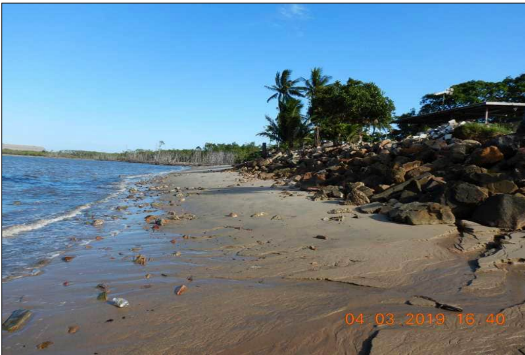
Figure 14: Retaining wall on the Dungeness Foreshore.
