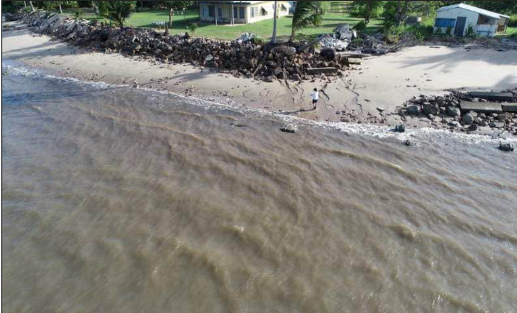
Figure 13: Aerial view of retaining wall on the Dungeness Foreshore.
