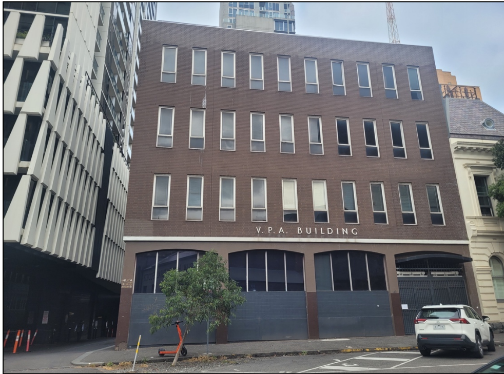
Figure 3 View of the subject site at 43 Mackenzie Street from Mackenzie Street.
