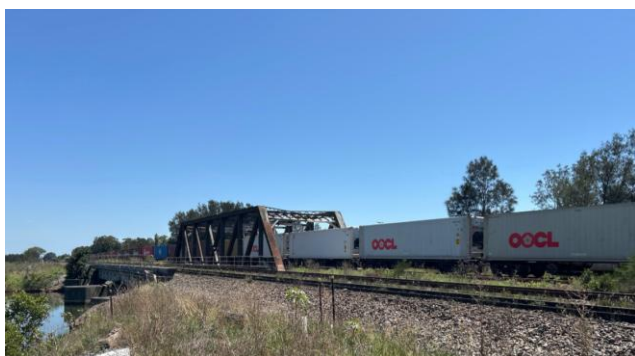
Plate 7: looking northeast from existing laydown area
