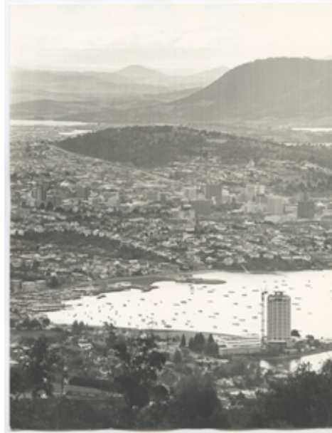
Wrest Point Casino under construction c1972 TAHO PH30_1_7384
