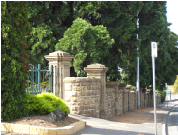
Former entrance gates and stone wall DPIPWE 2011
