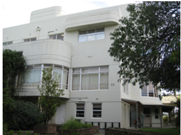
Rear elevation of the Riviera Hotel DPIPWE 2011
