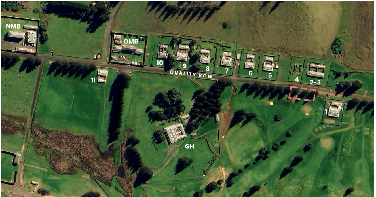
Figure 1: Aerial view, the Golf Club Workshop, subject of this proposal marked by red dashed line, located on Quality Row and adjacent to No. 1 Quality Row. (Source: Google Earth Pro and MAXAR Technologies 2023, modified by Purcell)
