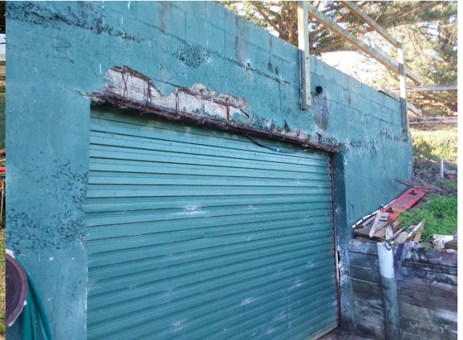
Figure 3: Entrance to Grounds Keeper's Shed. (Source: Purcell)
