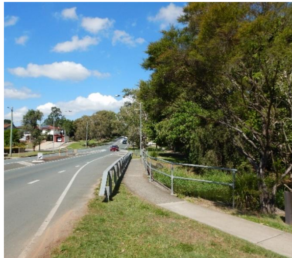
Figure 15: OGR-04 showing the culvert over Freshwater Creek, looking south. A grey headed? flying fox colony was identified approx. 50m to the west/upstream (to the right of the picture).
