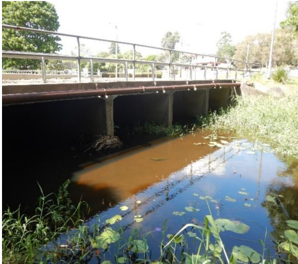
Figure 16: The Freshwater Creek Culvert will be widened. There is a limited potential for early historical fabric to remain in this area.
